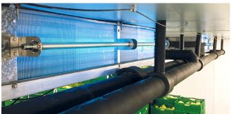
**sterilAir**<sup>®</sup> offers a powerful and environmentally friendly solution. Our UVC installations sustainably prevent build up and growth of biofilm. Clean coils keep energy consumption of the cooling unit constantly low. The slats remain hygienically flawless, cleaning effort and frequency decrease significantly - a considerable cost saving in operation and maintenance.
