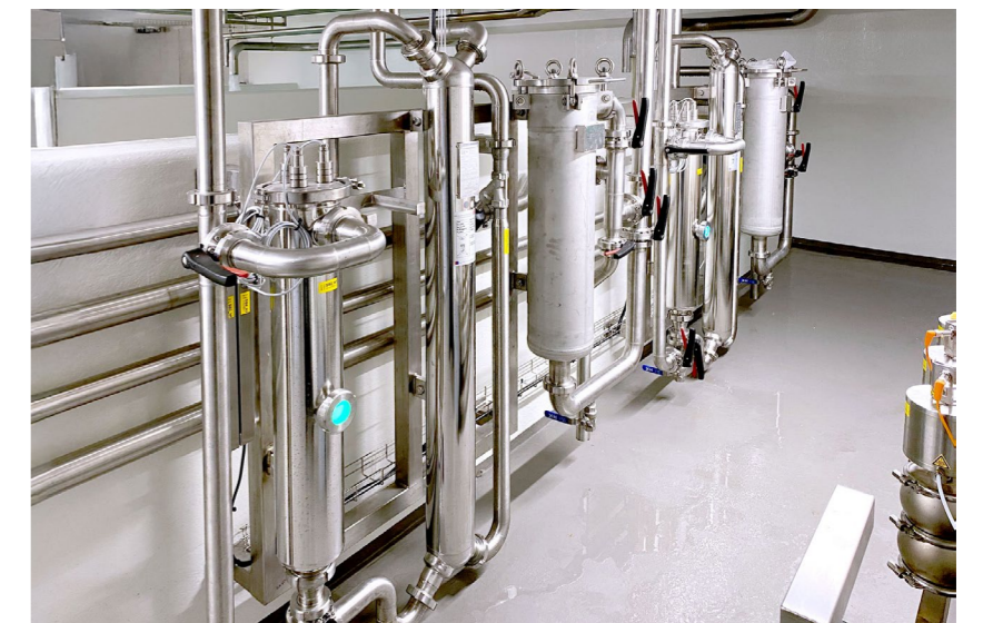
sterilAir AQD-ST reactors for UVC sterilisation of brine
