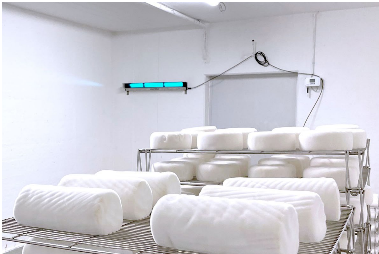
During the maturing of the soft cheese specialties, mould spores in the air are inactivated with a sterilAir wall emitter.
