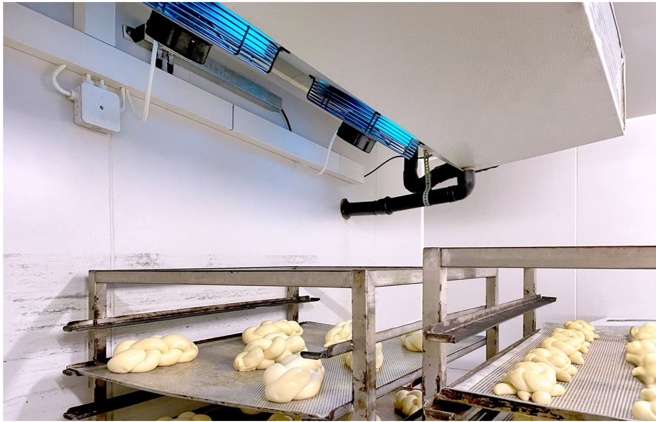
UVC disinfection in an air cooler ensures clean cooling coils and safeguards the air quality in the cold room
